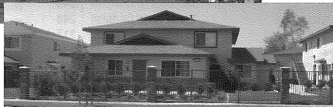
Rialto's troublesome Willow-Winchester condos (above) contrast with the rehabilitated units in Citrus Grove (below).
