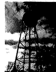
Elevated Storage Tank
