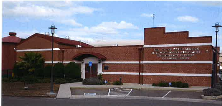
The Railroad Water Treatment and Storage Facility
