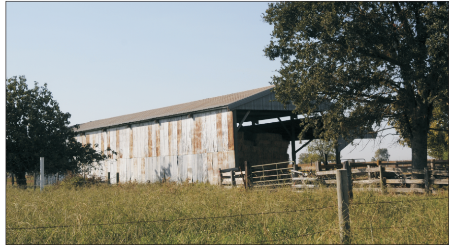
View of the Barn near the south end of Rau Road.
